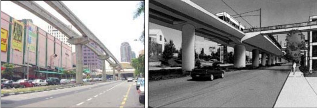
Figure 3.6—Monorail has the lowest impact of any elevated rail system. Notice the difference in shadowing effects between monorail and light rail aerials (Kuala Lumpur guideway (right), Projected Seattle light rail aerial (left)). Source: Monorail Malaysia/ Sound Transit.
