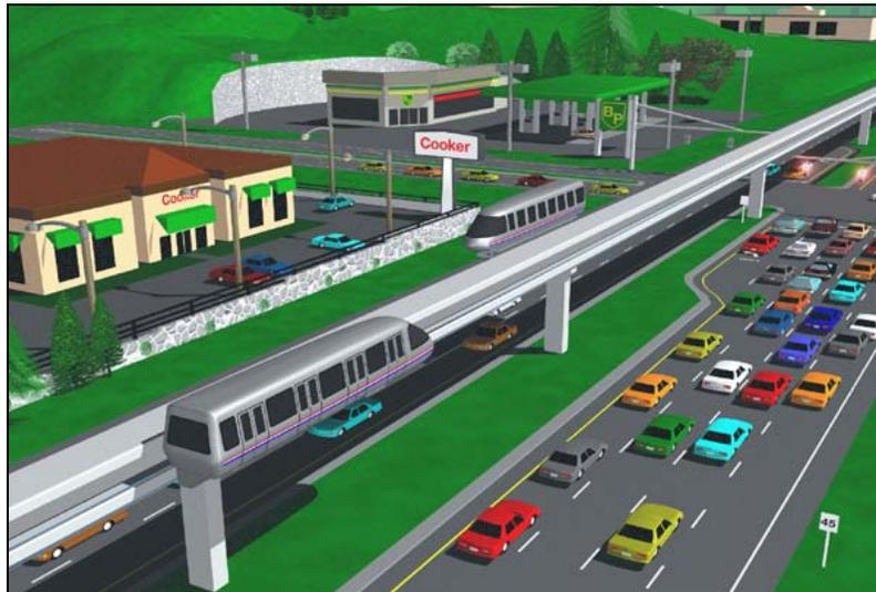
Figure 1.4--Owen Transit cantilevered monorail. Source: The Monorail Society
