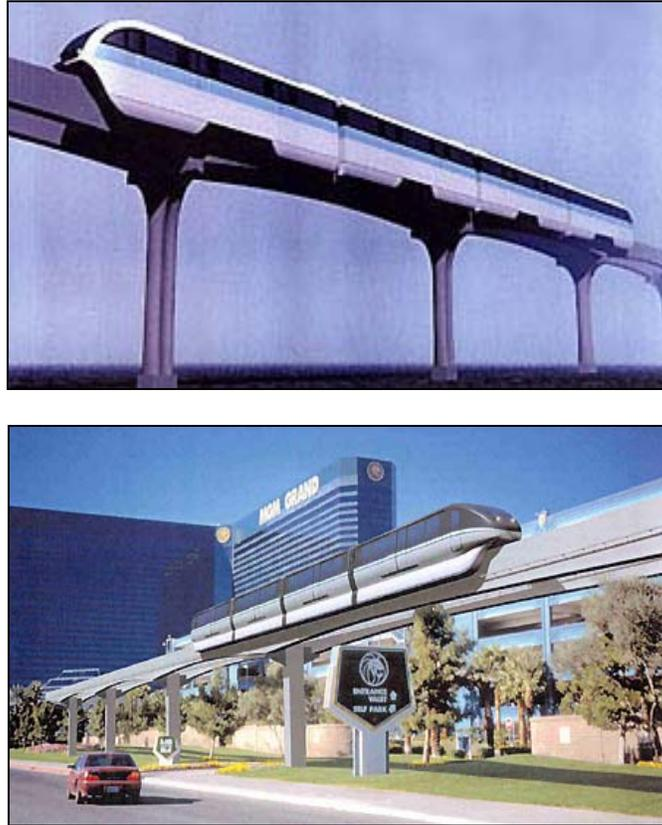
Figure 2.5—Two modern monorail aerial structures. Proposed Hitachi for Kuala Lumpur (Top) and Bombardier for Las Vegas (Bottom) The Bombardier aerial structure is the narrowest and most visually appealing of all the transit monorails mainly because trains are narrower than the competition and have a maximum gross axle load of only 8 metric tons.
