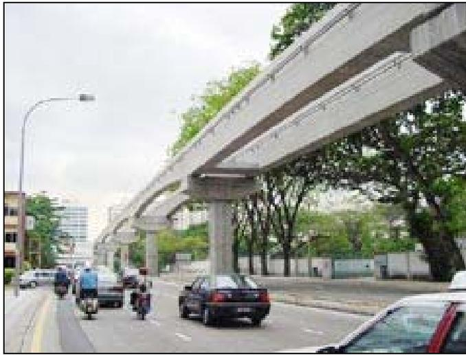
Figure 2.4—Kuala Lumpur monorail guideway has both straight (foreground) and arched (background) segments.
